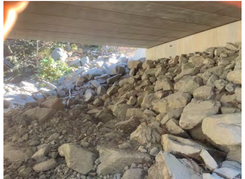
Left Bank Abutment when facing downstream
