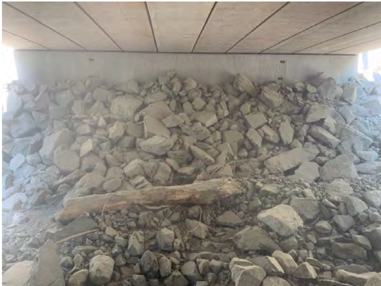
Right Bank Abutment when facing downstream
