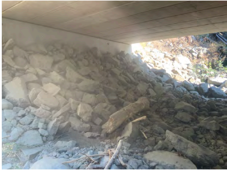
Right Bank Abutment when facing downstream
