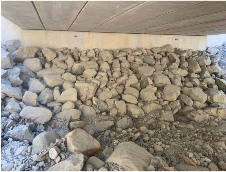
Left Bank Abutment when facing downstream
